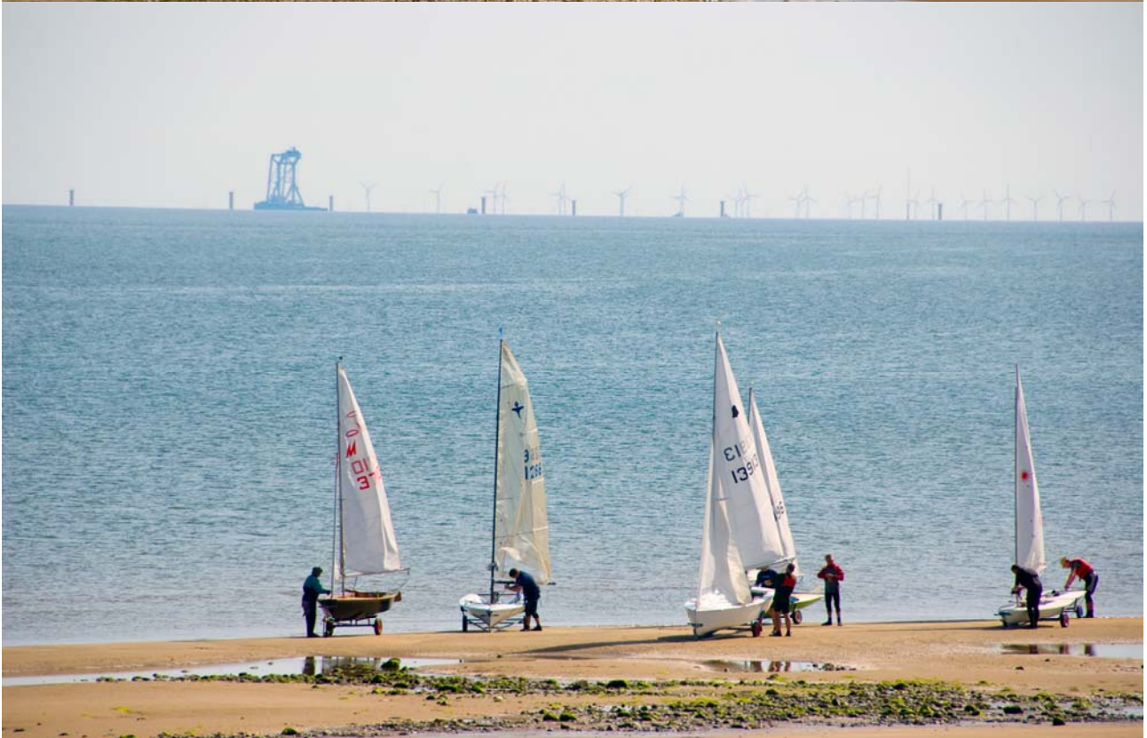
Views of the Rhyl Flats construction from Llandudno Promenade with North Hoyle windfarm in the background – 16 miles away.
